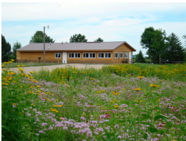
(South) Enclosed Shelter $50/per day Rental – Water Hydrant–Electricity–Air Cond.–Rest Rooms–Seats 64
